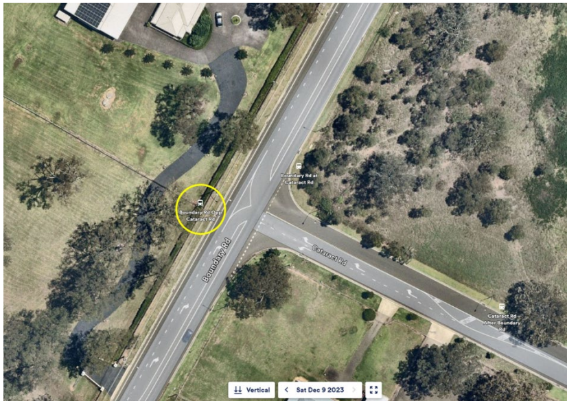
Figure 1 - Existing Northbound Bus Stop in Boundary Road
